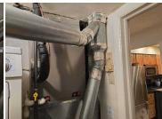
14. Maintenance Item TPRV and Drain Tube: Missing - TPR Valve drain tube is missing. Recommend drain tube be installed and should not be more that 6 inches from the floor. This is to help prevent scalding, by hot water, of anyone that may be nearby should the pressure relief valve open to release excess pressure/water buildup in the hot water heater.
